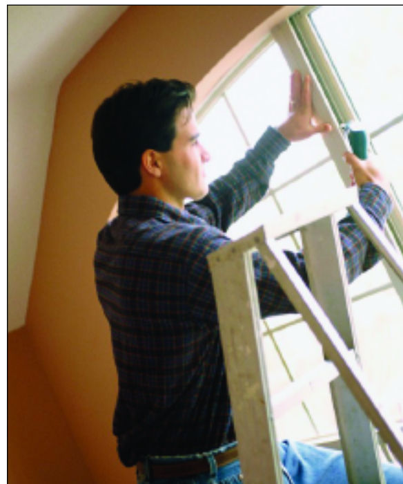
Properly sealing windows will reduce drafts and help lower heating costs.
